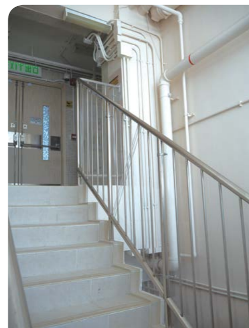
Replaced with non-slip floor tiles and increased the height of the fence to prevent incident 更換防滑地磚及加高圍欄，預防意外發生
